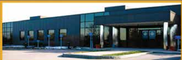
CNSE PHOTOVOLTAIC MANUFACTURING AND TECHNOLOGY DEVELOPMENT FACILITY (CNSE MDF) - ROCHESTER
